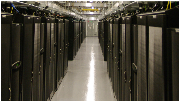
Massachusetts Green High Performance Computing Center (mghpcc.org)
